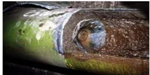
D 500 pipe in the cleaning phase
