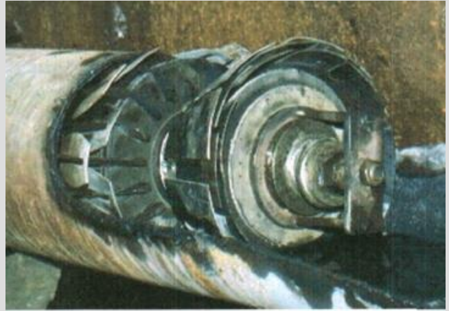
Introduction of the generator to the pipeline
