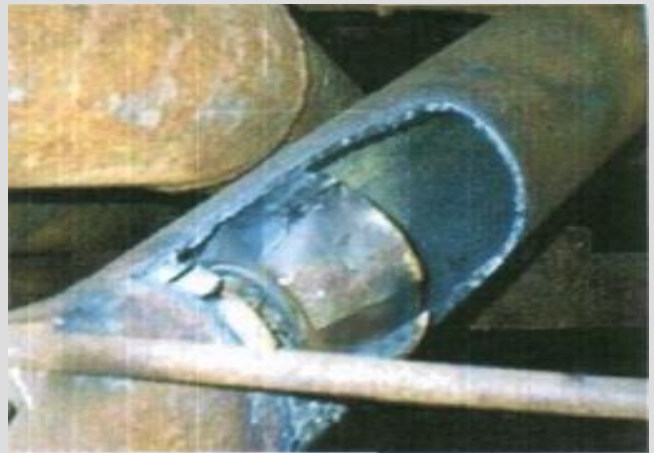
Making an inspection hole to remove the generator
