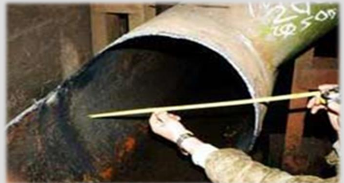
The pipe after cleaning using a cavitation generator.
