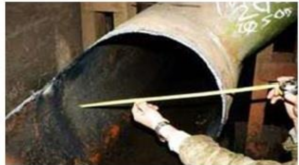
Example of a D 500 mm pipe after cleaning
